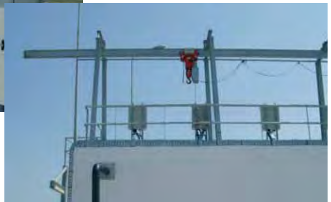
Electric Chain Hoist with electric trolley Type 66/04 AKE capacity: 5 t installed in a sewage plant in Tunisia
