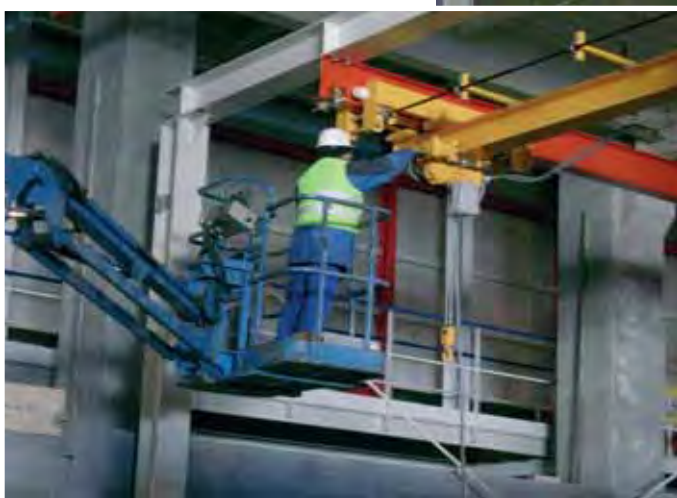
crane installation
